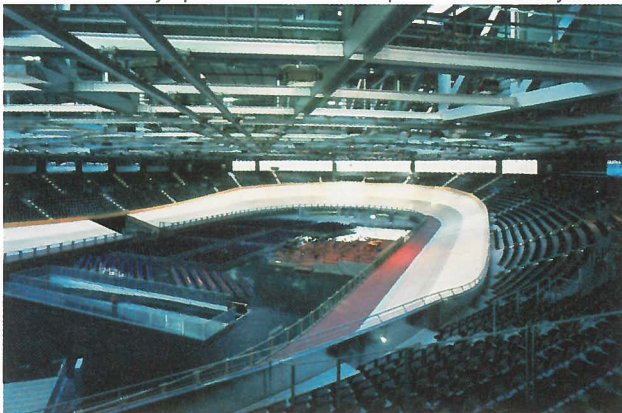
32. Interior of Olympic Velodrome and exposed structural system
