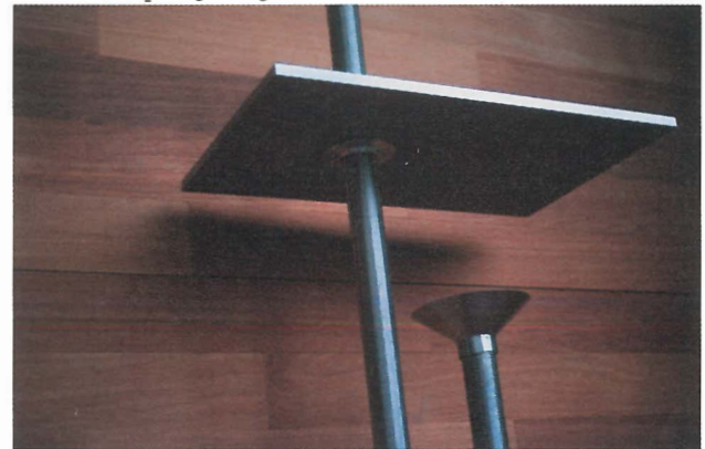
44. Interior lighting along corridor
