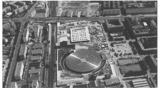
4. Aerial view of construction: Olympic Velodrome and pool, Berlin
