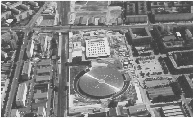
29. Aerial view, construction, Olympic Velodrome and pool, Berlin
