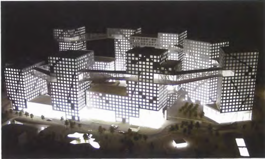
(Fig: 33) Steven Holl, Hybrid Building, Beijing (2003-09). This conglomeration of eight, medium-rise towers, linked by aerial bridges, accommodates 2,500 people in a 'loop' around a retention lake, a cinemathèque and hotel. This compound is flanked by a series of artificial green earthworks, known as 'mounds', ostensibly representing the four ages of man. The entire complex is heated by 100 foot deep geothermal wells. The aerial bridges accommodate such facilities as a swimming pool, a fitness room, a cafe and a gallery. As the architects put it, the overall aim was to "express a collective aspiration rather than towers as isolate objects or private island in an increasingly privatized city."
