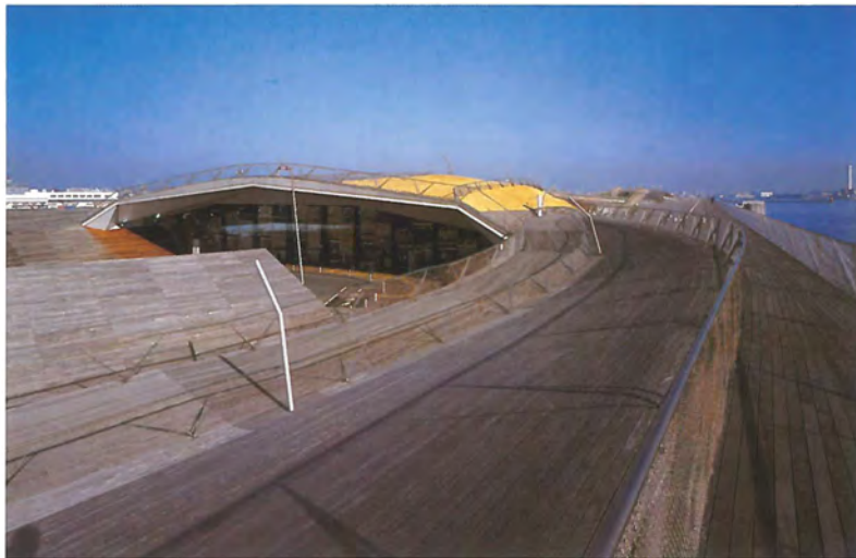
(Figs: 42 - 43) Alejandro Zaero Polo and Farshid Mousavi (Foreign Office Architects) Yokohama Ferry Terminal, Japan (2002) this terminal is a quintessentially hybrid megaform comprising, in addition to its basic terminal facilities, a promenade-pier and public park on top of a large reception space and auditorium. While this is an imminent demonstration of parametric method, the framed structure sustaining the terminal is transformed in section while maintaining its axial order and geometrical integrity.
